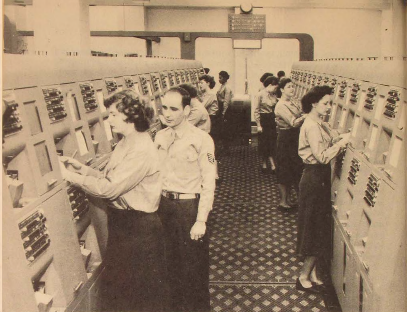
The switching center in the Pentagon, a part of the United States Air Force's new nationwide, push-button, high-speed telegraphic network that links 118 stations in the United States into the Air Command Communications Network. The new system, which requires only five switching centers to replace the twenty-eight centers formerly in use saves four hundred operators and, eventually, more than one million dollars a year.
